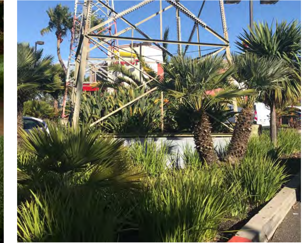
EXISTING POWER LINE TOWER W/ PLANTING AND ACCENT LIGHTING
